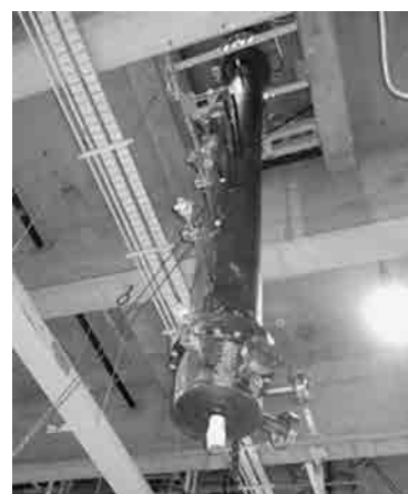
Fig. 5 Equipment such as fluoridation furnace
