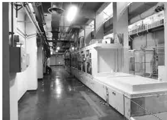
Photo 9 External appearance after No. 11 and No. 12 lead cells removal
