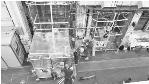
Photo 5 Isolation tent for contamination control
