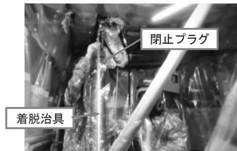
Fig. 11 Picture of removal work of pressure tube plug
