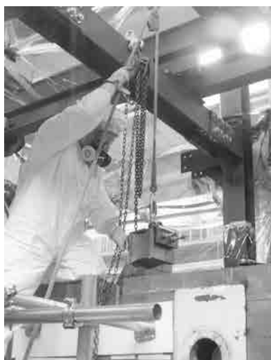
Photo 7 Removal of lead block
