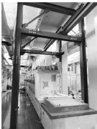
Photo 6 Lifting frame for isolation tent
